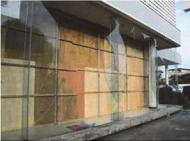
Photo 1 Earthquake Damage Example of Glass Screen System of Low-rise Steel Frame Building<sup>2)</sup>
