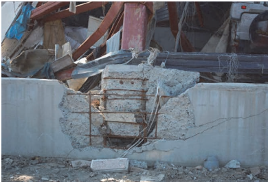
(c) 0-1-B 柱脚 (全体)
